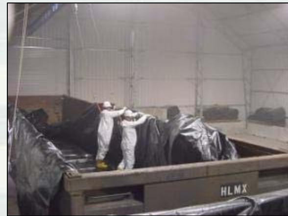
Workers preparing railcar for offsite shipments of radium contaminated soils and debris for the Shattuck Superfund Site, Denver, CO
