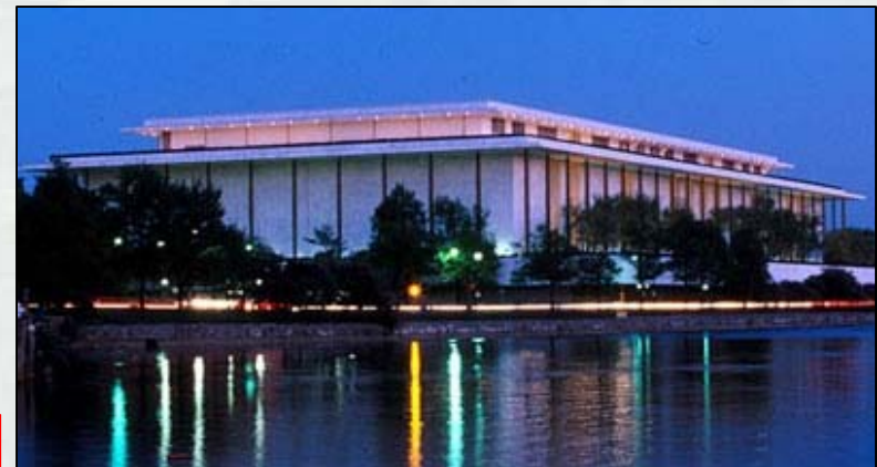
Security upgrades at the Kennedy Center
